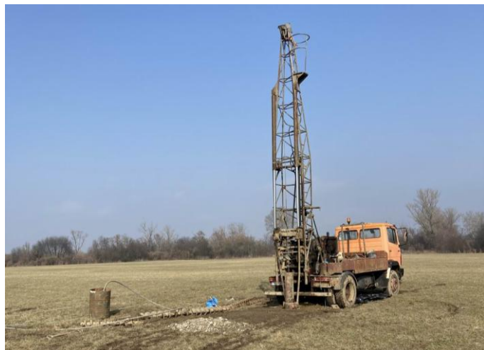
Drilling of piezometers to collect water and soil samples.
